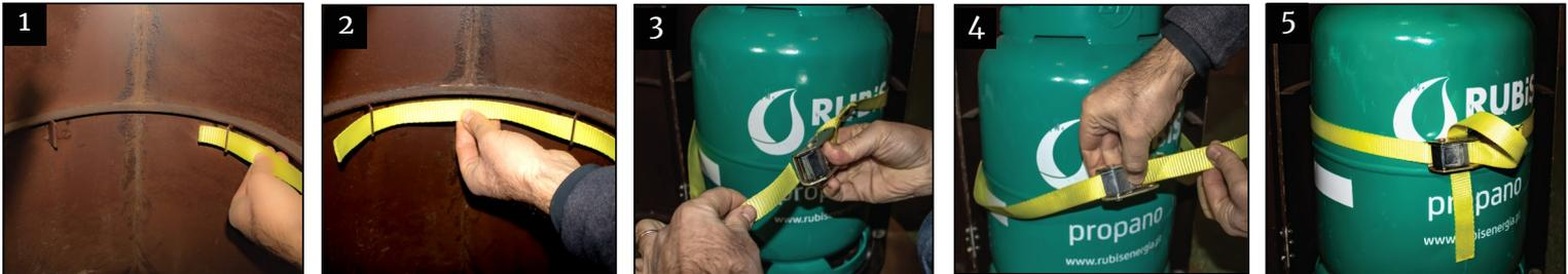
Photo scheme for strapping and gas cylinder placement
